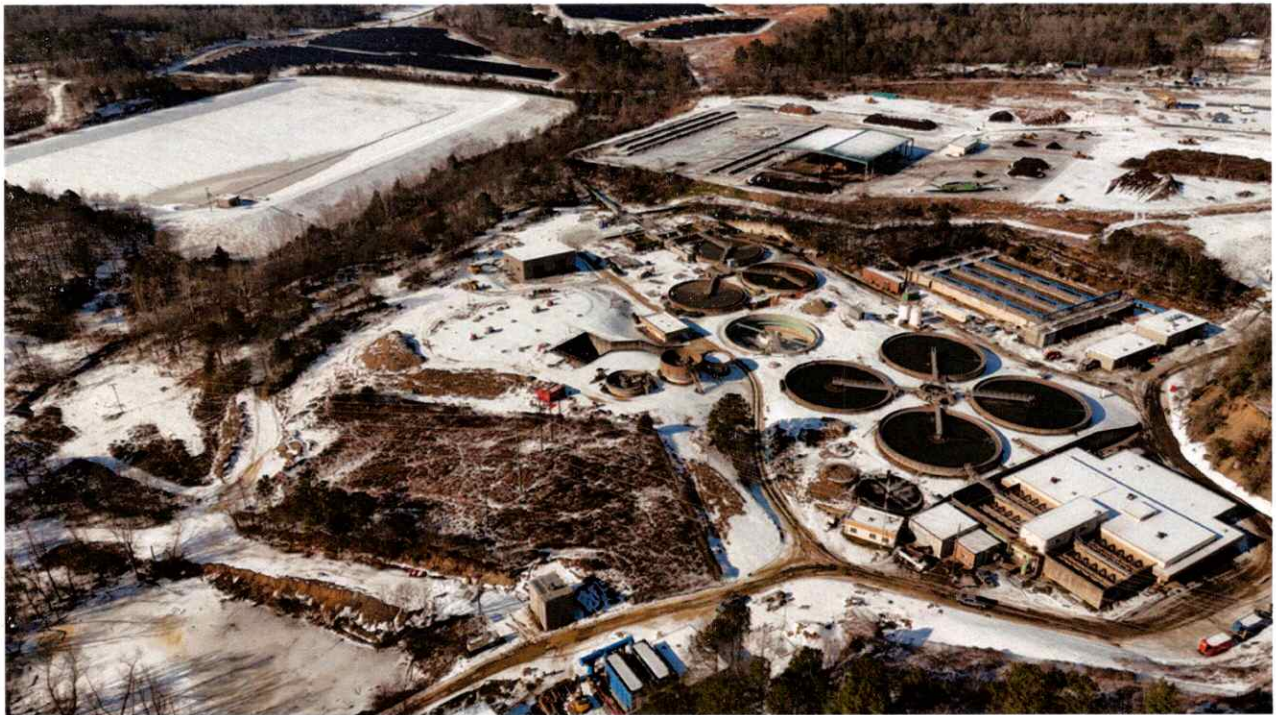
Davidson Drive WWTP Improvements
